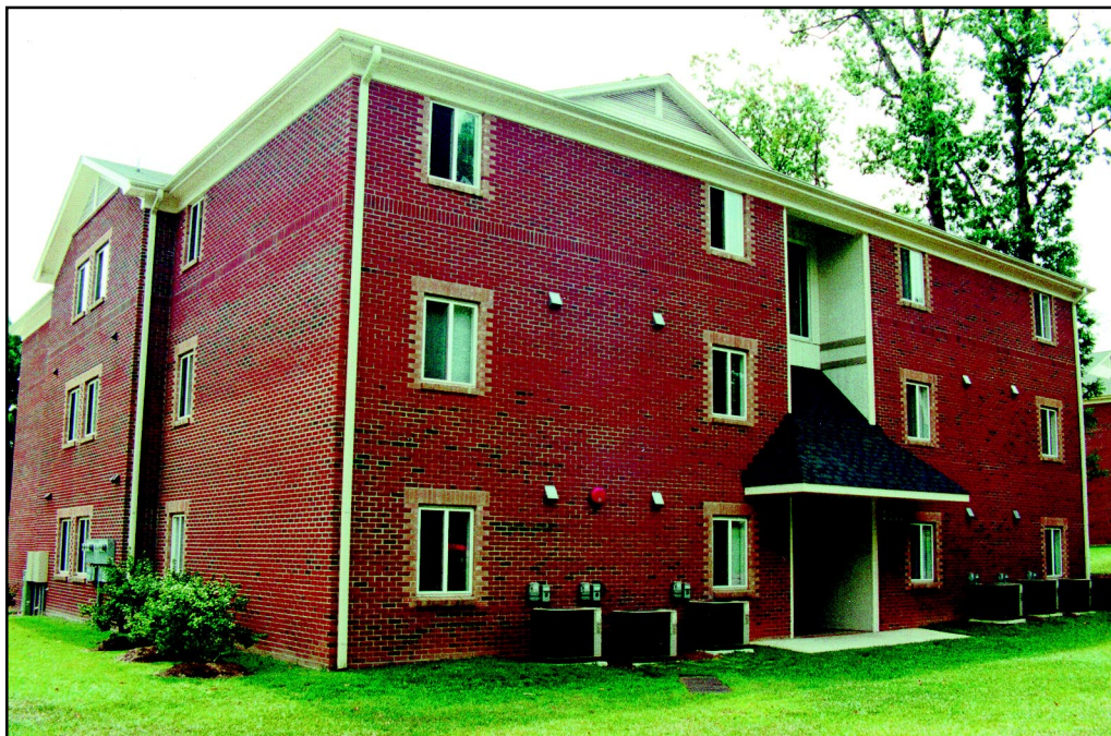
Three-level student apartments in Greensboro, N.C., use energy recovery ventilation systems to save energy.
